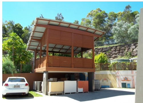
The external staff area, with its curved roof and solar panelling
