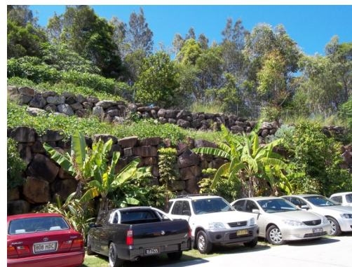
The back of the property, with its large retainer walls, and lots of potential!
